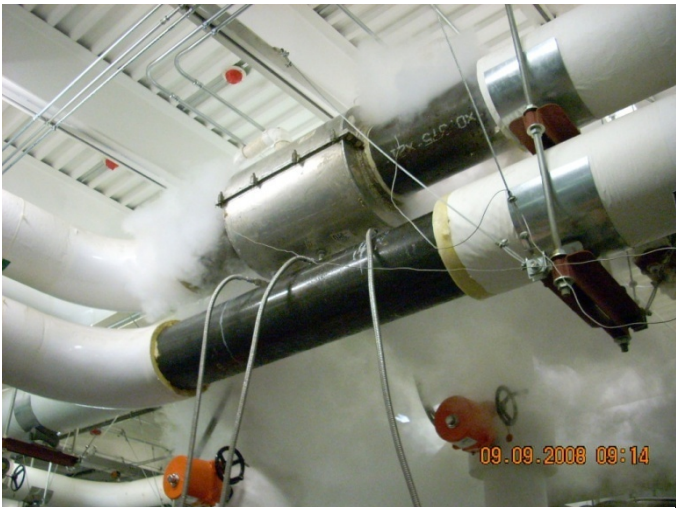
Freezing 16" Chilled Water line for Valve
