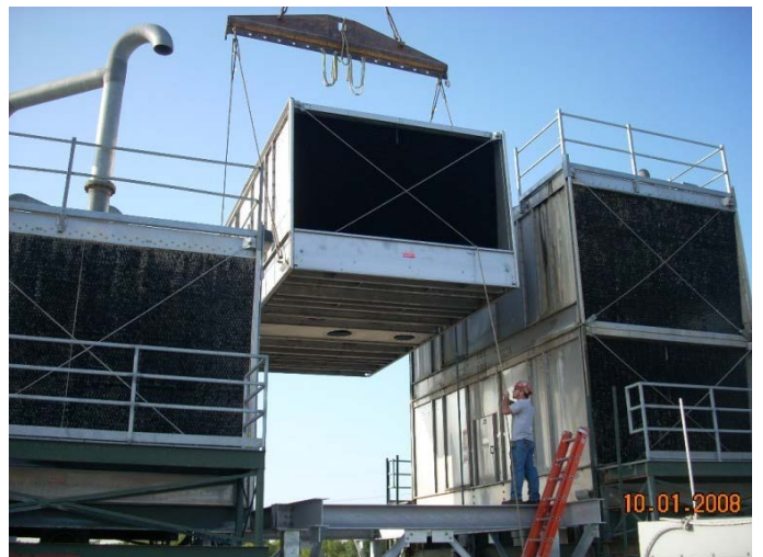
New Cooling Tower Installation
