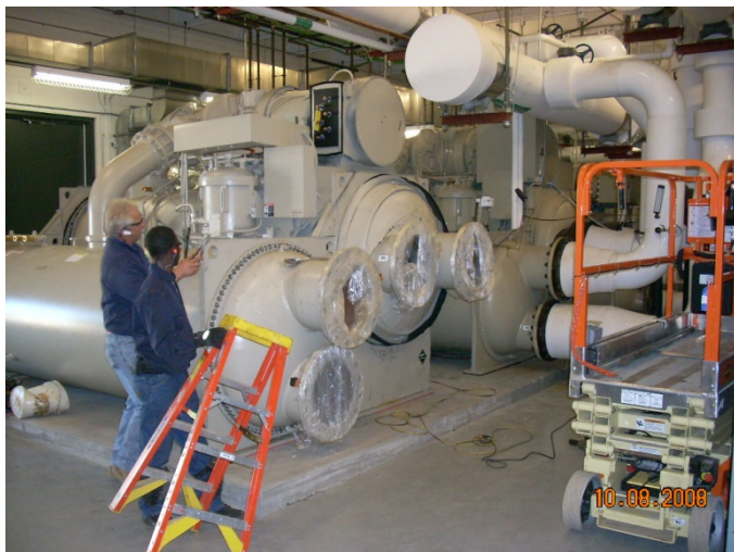
Installation of 900 Ton Chiller
