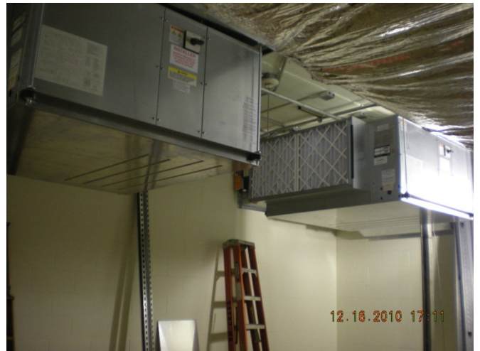
Installation of new Liebert CRAC Unit
