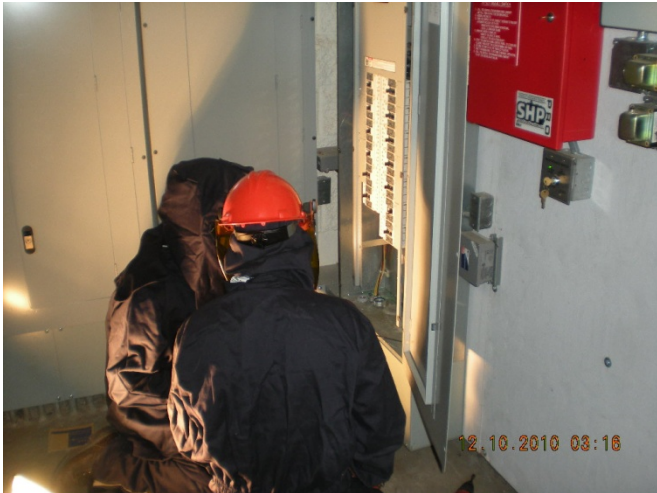
Breaker Replacement in HVAC-1
