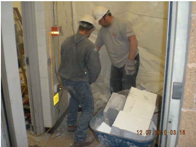
Demo of existing CMU Wall
