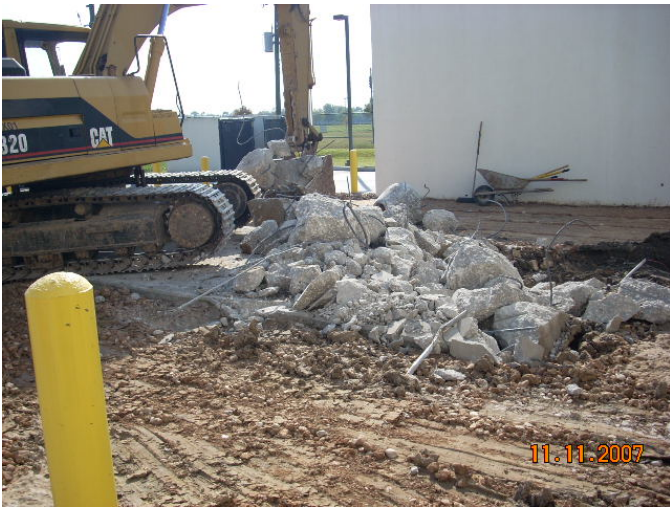
Removal of Existing Generator Pad
