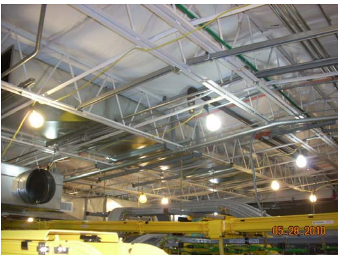
Installed Main Trunk and Branch Runs
