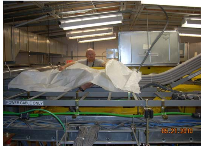
Protecting network prior to duct installation
