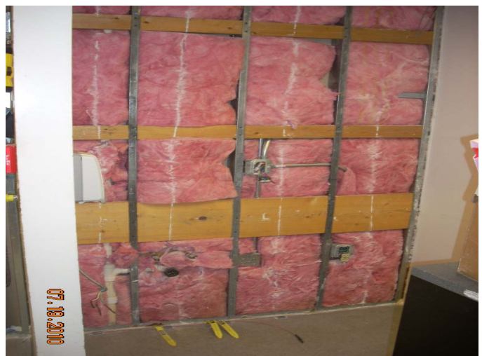
Installed Framing and Insulation
