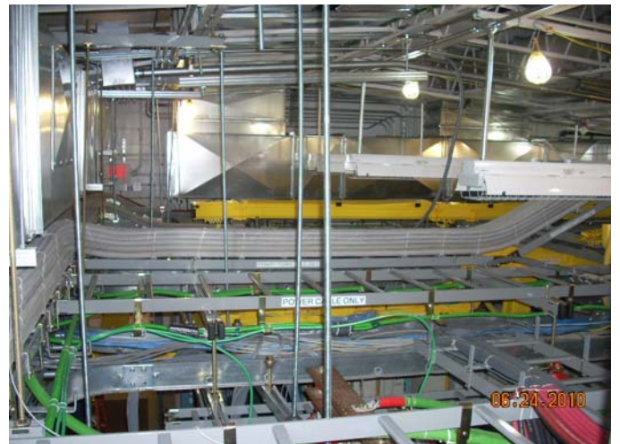
Temporary lights for duct and seismic work
