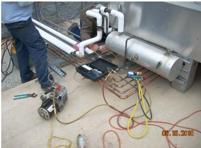
Installing refrigerant lines
