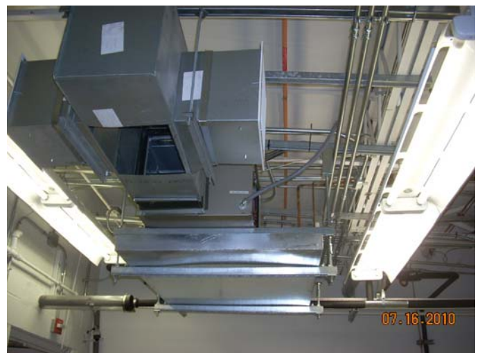
New ductwork installed for airflow above switch
