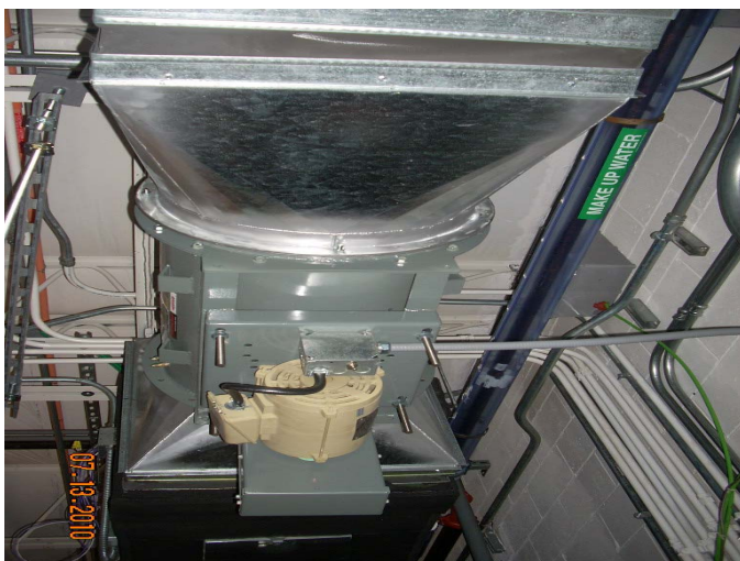
New in-line fan installed above live switch
