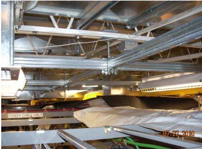
New Aux framing and protection above switch
