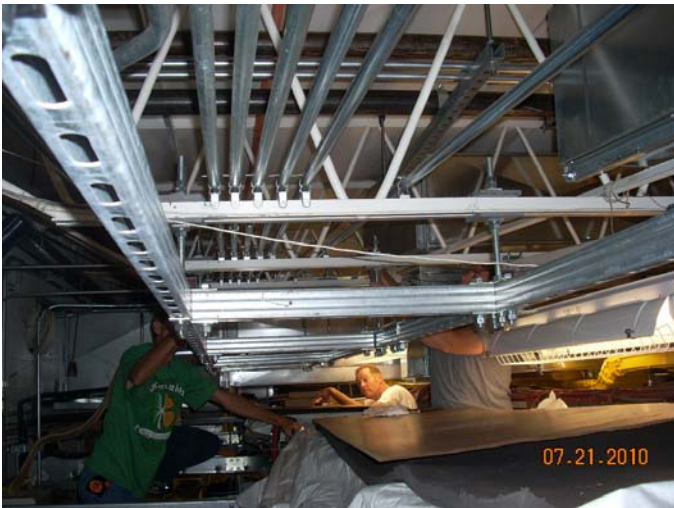
Installing New Auxiliary Framing
