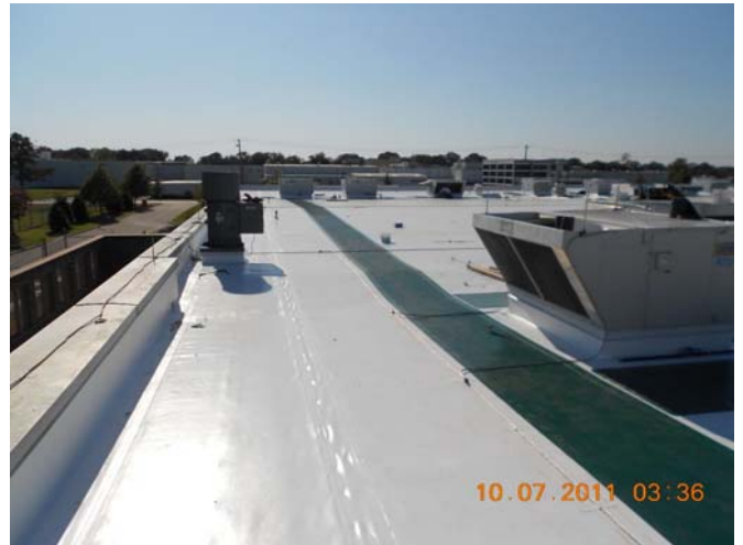
Completed Roof, Walk Mats & Lightning Protection
