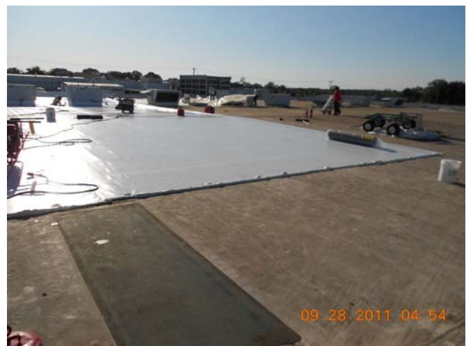
New Sarnafil Roofing Overlay of Existing Roof
