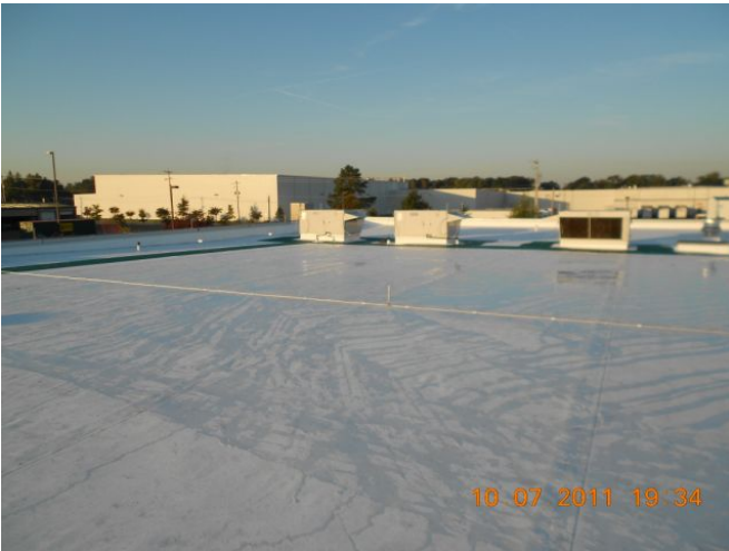
Completed Area after First Rain
