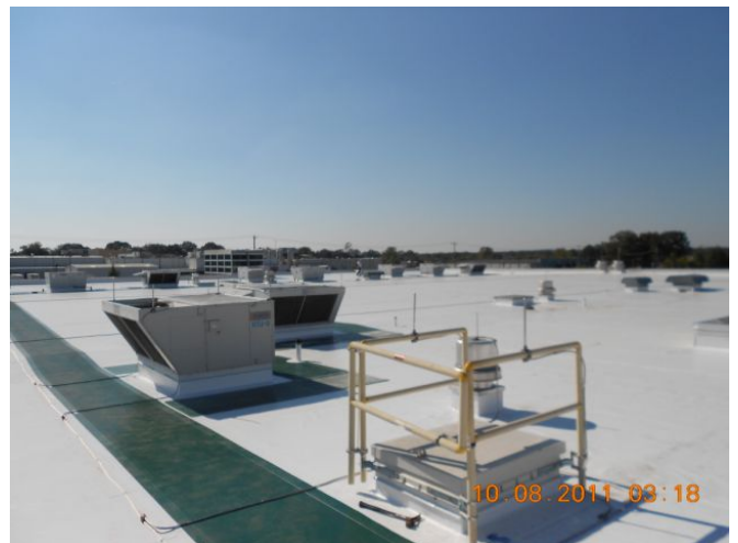
Completed Roof, Walk Mats & Lightning Protection
