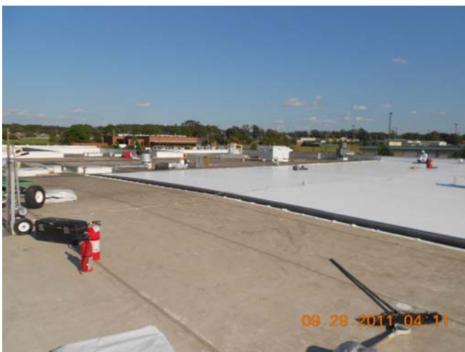
New Sarnafil Roofing Overlay of Existing Roof
