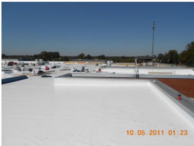
Completed Roof Area, Coping & Lightning
