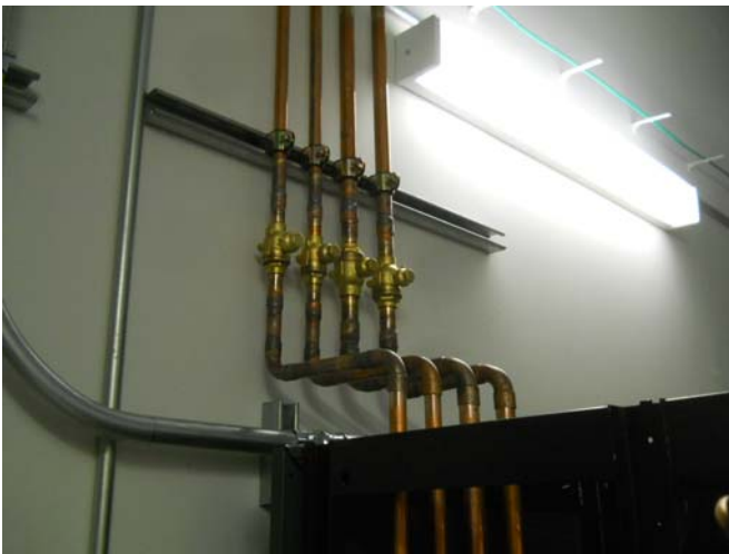
Refrigerant Piping Ready to Braze
