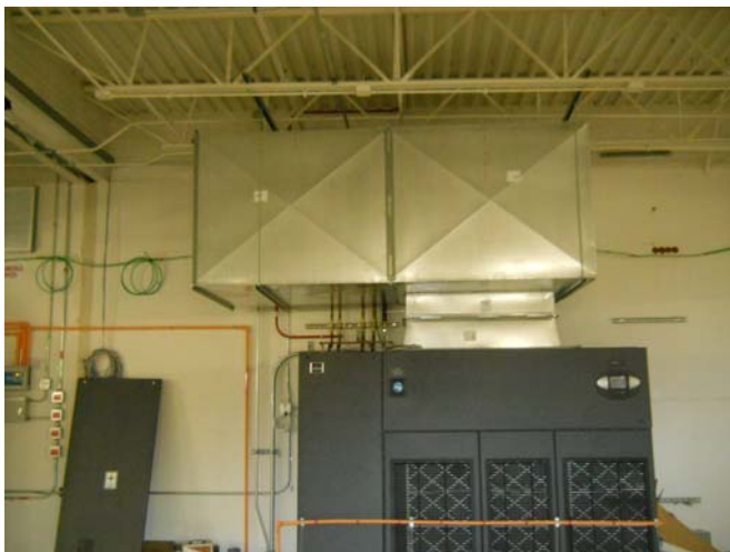
New Duct on CRAC Unit #21
