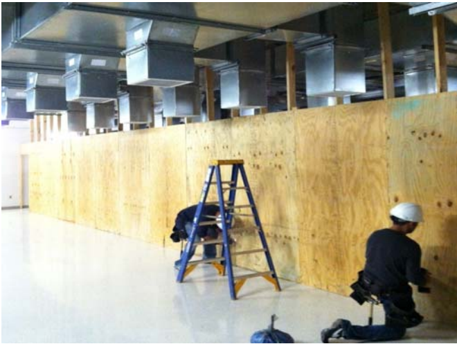
East Wall Dust Protection Installation
