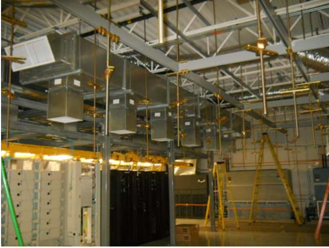
Installing Cable Tray Racking
