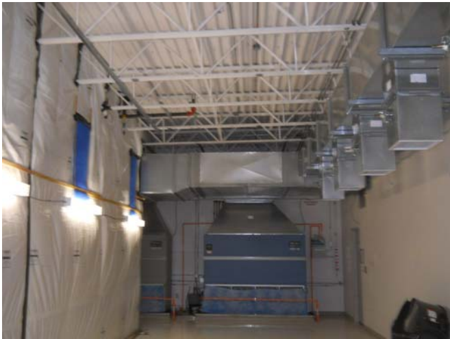
Ductwork Removal Complete
