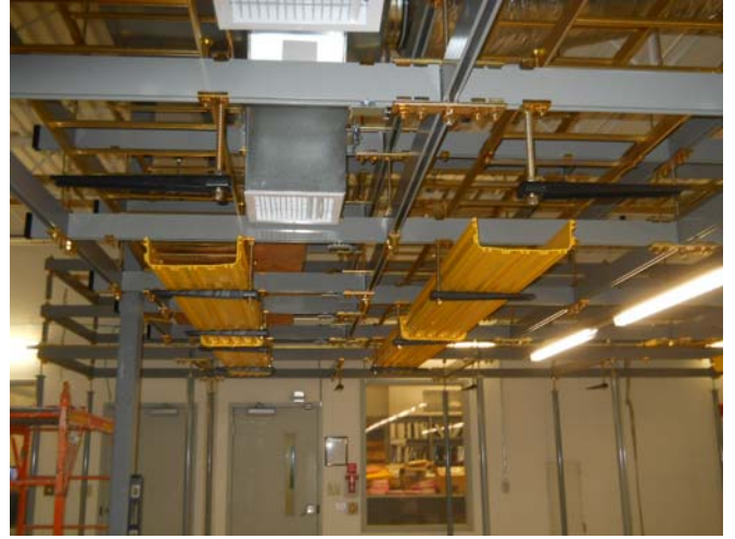
Installing Fiber Duct
