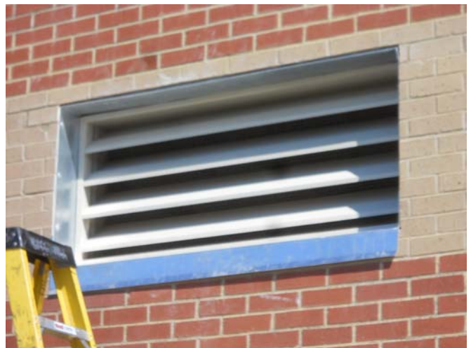
Louver Installed
