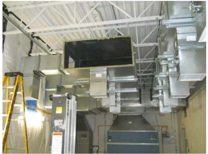
Removing Existing Ductwork
