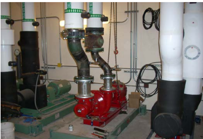
Chilled Water Pump Installation
