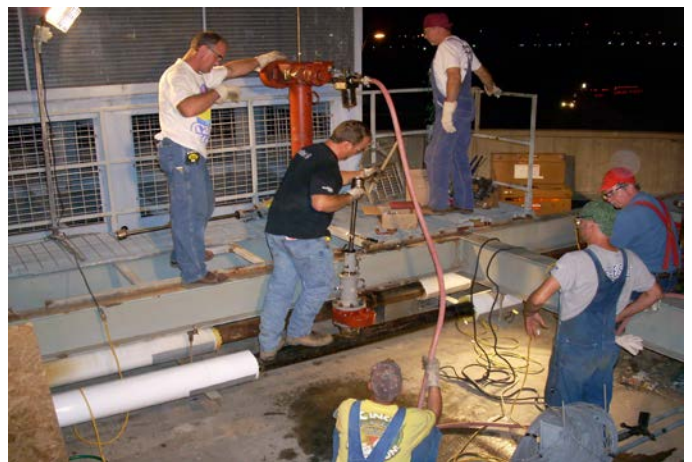
Installation of Stopple Valve
