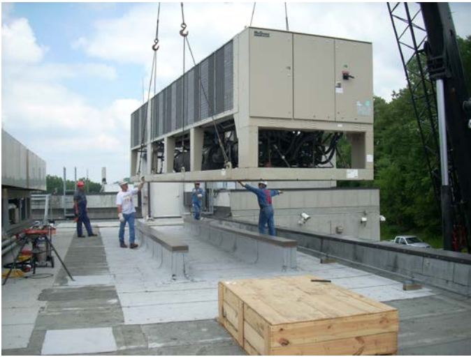
New Chiller Installation
