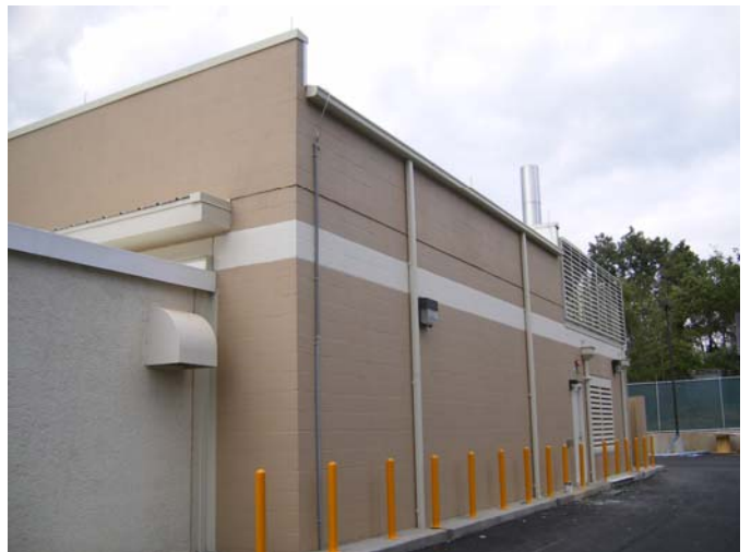
Completed Building Expansion
