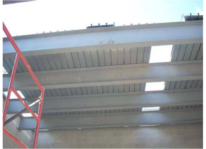
Structural Steel and Roof Decking
