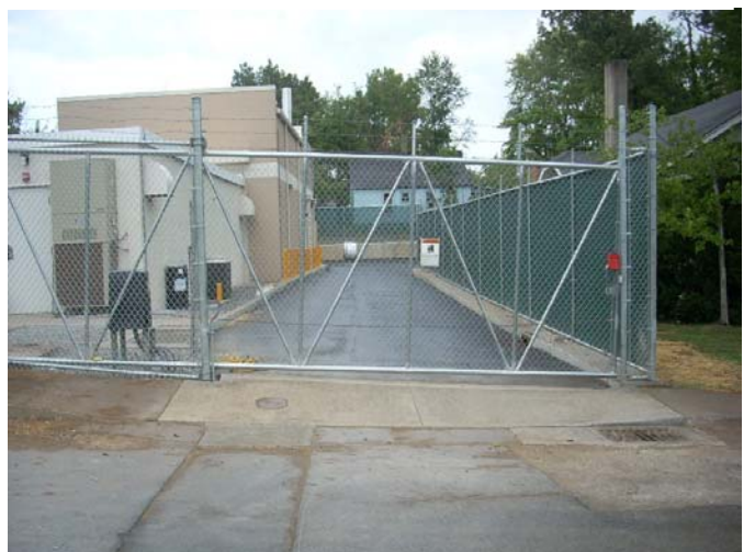
New Asphalt Drive, Retaining Wall & Gate Operator
