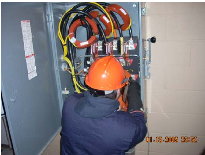
Installing BAS in Manual Transfer Switch
