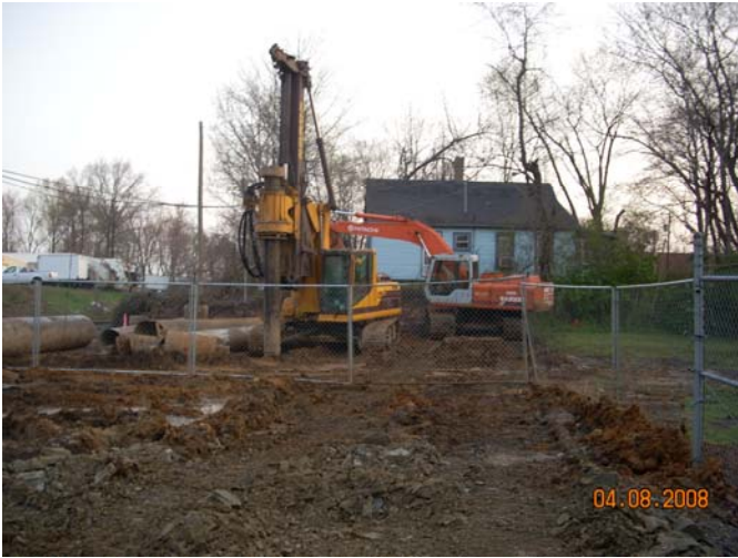
Drilling Foundation Piers
