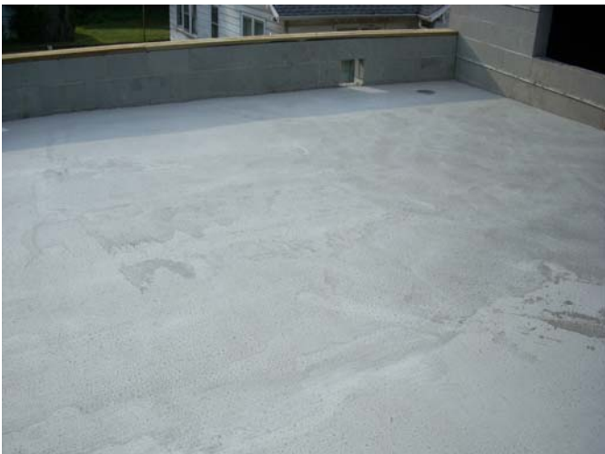
Completed Concrete Roof Deck
