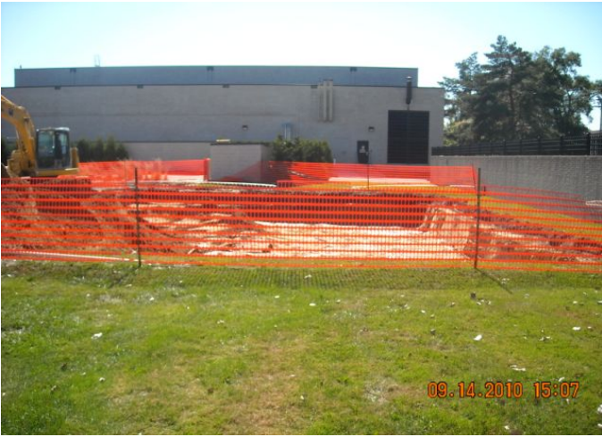
Generator Pad Excavation and Security Fence
