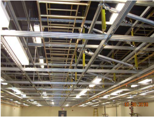
Installation of Auxiliary Framing System in Multiple Critical Rooms
