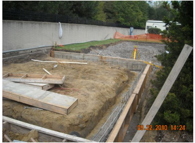
New Generator Pad Footings & Forms
