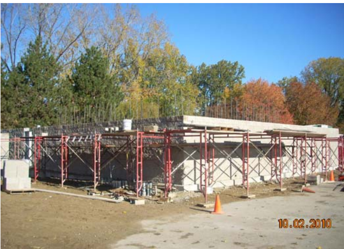
New Generator Screen Wall Construction
