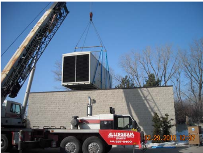
Setting Enclosure over Generator
