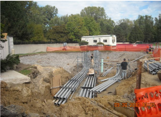
Underground Electrical Conduit Installation
