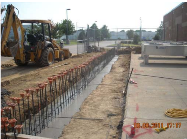
East Side Footings
