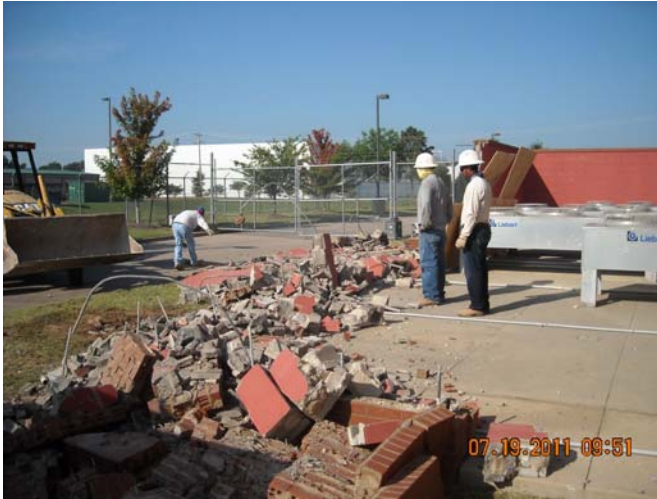
Demolition of West Wall
