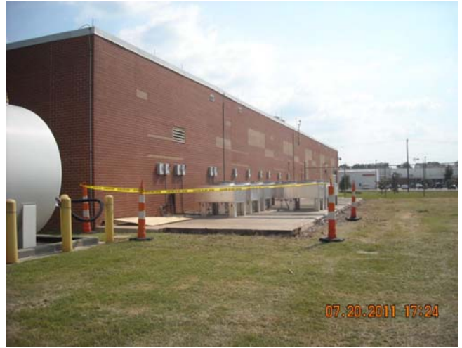
Safety Cones & Tape in Place
