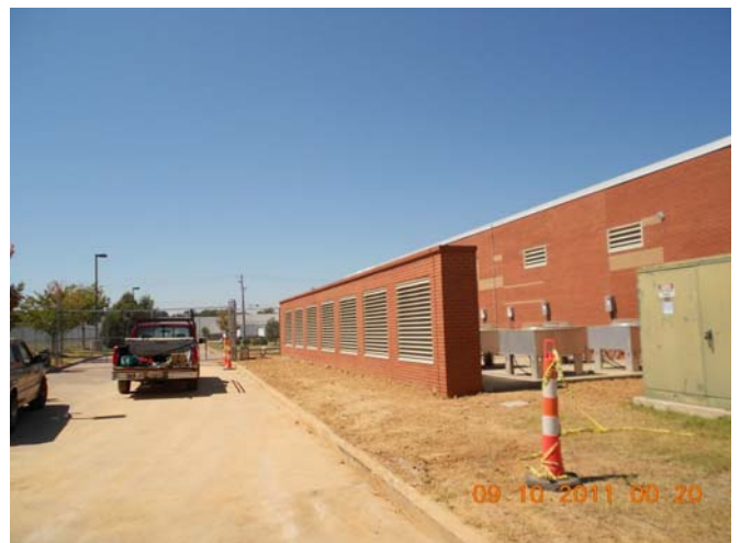
New East Wall Constructed and Louvers Installed
