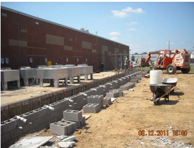
Construction of New West Wall
