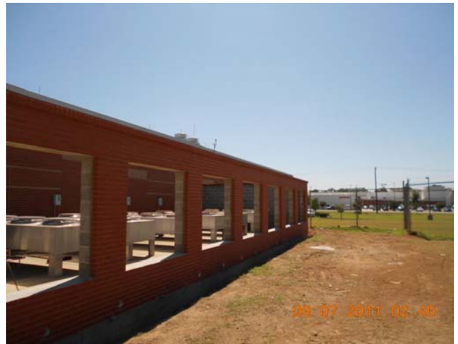
West Wall Nearing Completion
